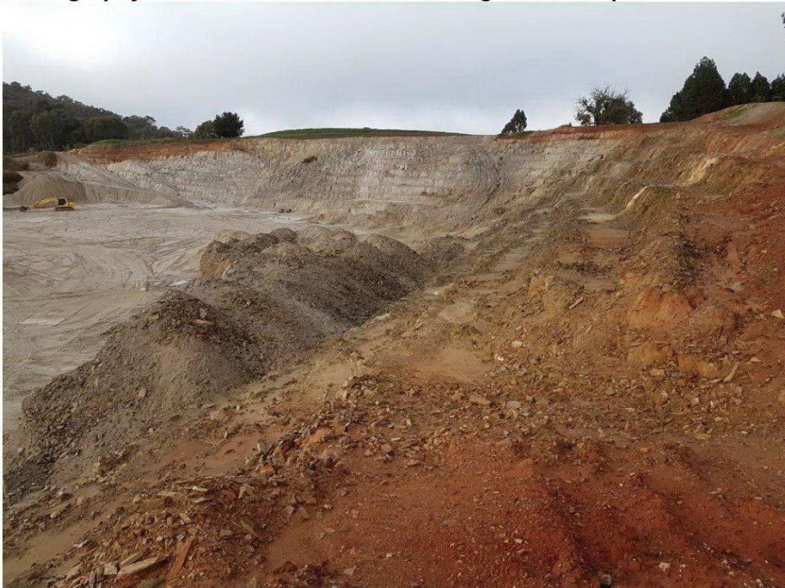
Photography 11: Stable batters and benching in current pit
